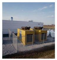
systems located outside a building are often exhausted directly out the top of the units.
