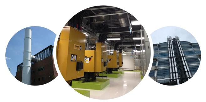
Generator exhaust systems for years have been fabricated from sections of schedule 40 carbon steel pipe that are field welded, then insulated to reduce surface temperatures.
