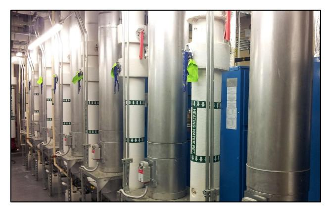
Proper product selection for Special Gas Vent exhaust systems for high efficiency boilers and hot water heaters can be a difficult process. There is a definite lack of detail provided by code, including International Mechanical Code, Uniform Mechanical Code, NFPA 211, and National Fuel Gas Code/NFPA 54.
